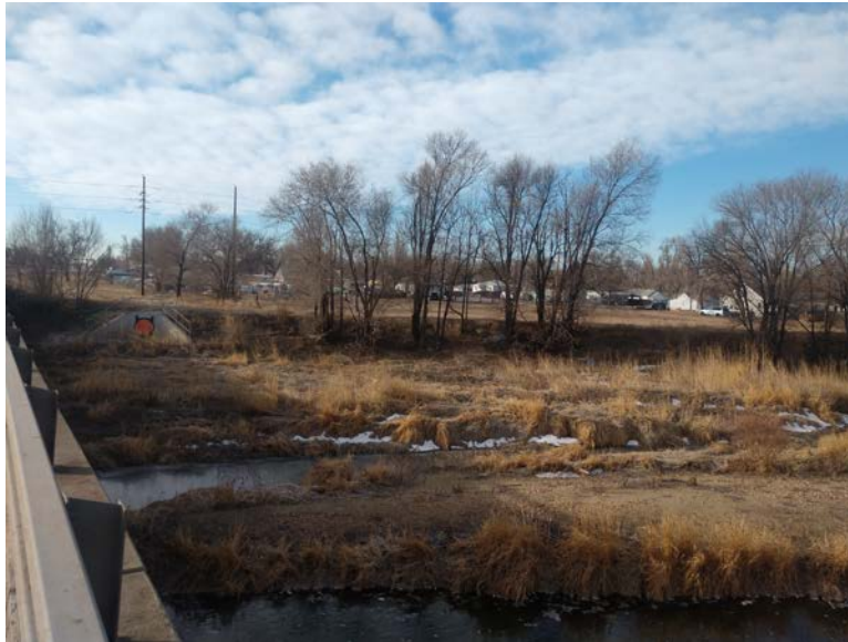
Figure 3 – Outfall Area from Highway 85 Bridge (Existing CDOT WQ Outfall on left)
