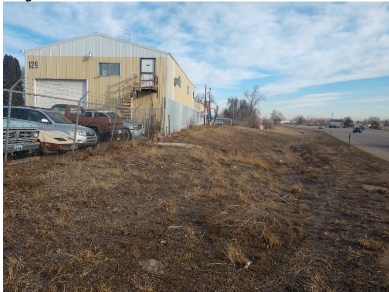
Figure 7 – CDOT ROW as viewed north from 12 th Street. Distance from property line to roadway varies from 40 to 75 feet
