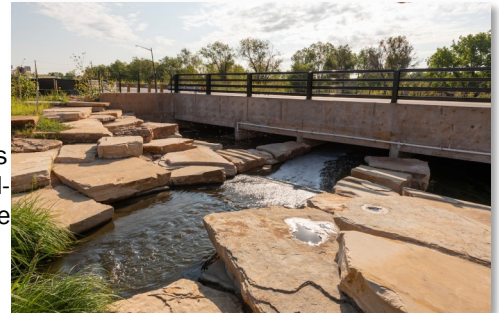
Sanderson Gulch Channel Improvements—Denver, CO
