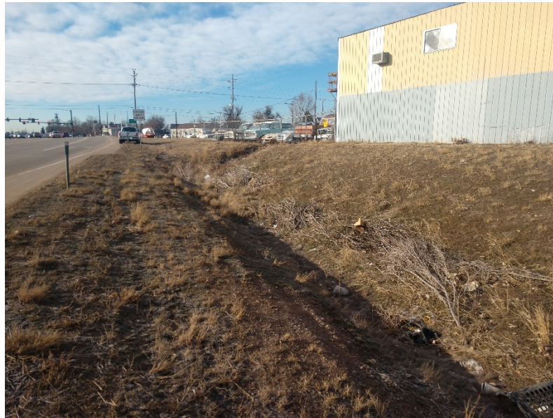
Figure 8 – Location of tightest clearance between Highway 85 and private property. Storm alignment must make 60 degree turn along approximate alignment of existing pictured swale
