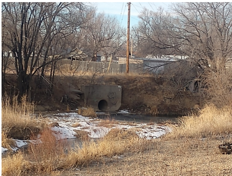
Figure 4 – Existing 48" Storm Outfall
